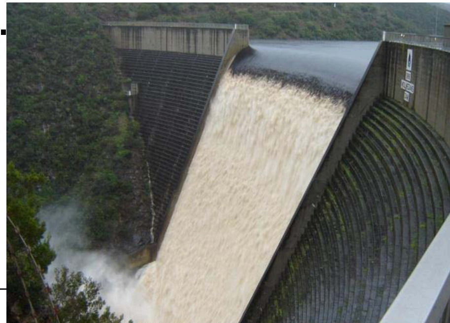
Wolwedans Dam. 3 Aug 2006 DWAF Hydro - Western Cape
